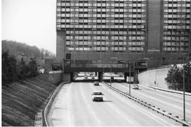
**FIGURE A.3.3.39.1 Air-Right Structure.**
