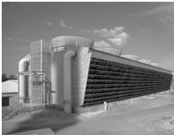
FIGURE B.1(e) Typical Induced-Draft Crossflow Water-Cooling Tower.
