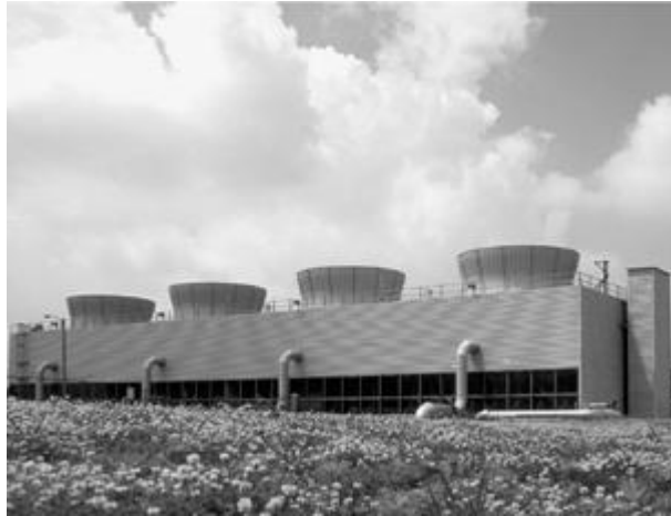
FIGURE B.1(d) Typical Induced-Draft Counterflow Water-Cooling Tower.
