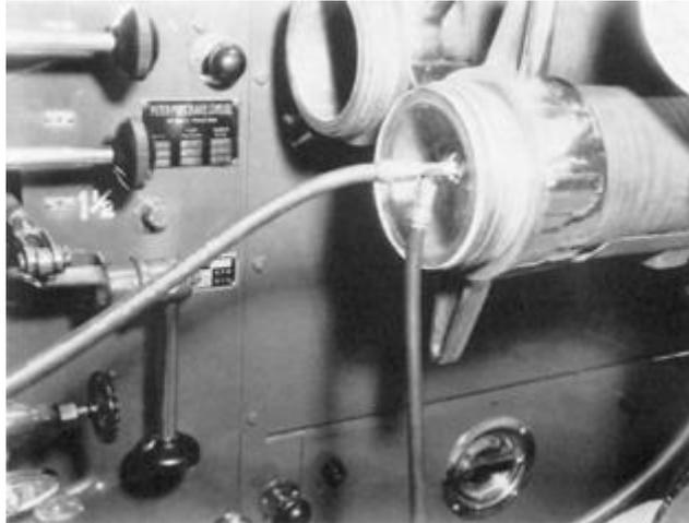
**FIGURE A.7.5.1 Plastic Test Disk for Pump Suction Hose. (Courtesy of San Diego Fire Department)**
